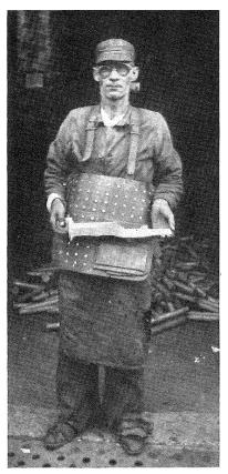
FIGURE I: Steel-bradded leather aprons are worn by casting grinders at the American Steel Foundries to protect the abdomen from vibrations
